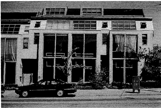
Figure 3b: Kitsun Townhouse project (Units 4-7) - 1987
