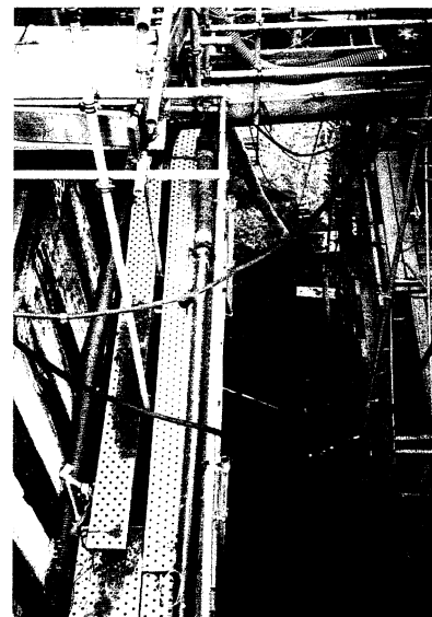
Picture 5 Placing LSS
