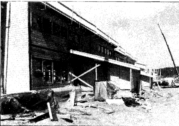
Fig. 15, 16, 17 Installation of elements
