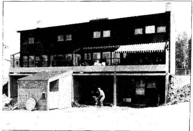
Fig. 26 The completed building
