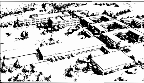
Figure 3. SMHI is the Swedish Meteorological and Hydrological Institute. There are laboratories and offices for a staff of 425 people. The institute is situated in the outskirts of Norrköping and is divided into a number of separate buildings, a large part of which are only 1 or 2 storeys. The most frequent type of window is larger than average, with a glass area of 0.96 \text{ m}^2 .
