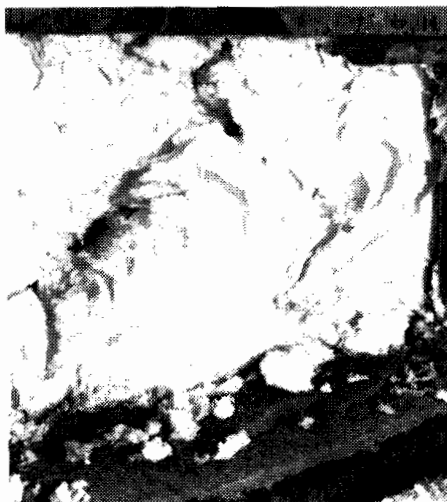
Figure 4: Fissures in urea-formaldehyde cavity wall insulation
