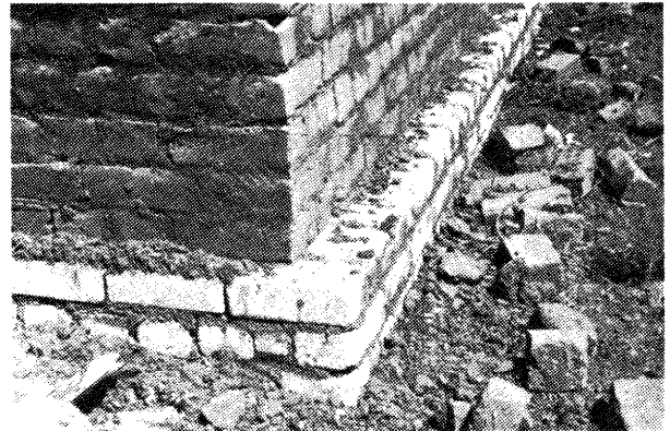
Fig. 3.3. Foundation and wall.
