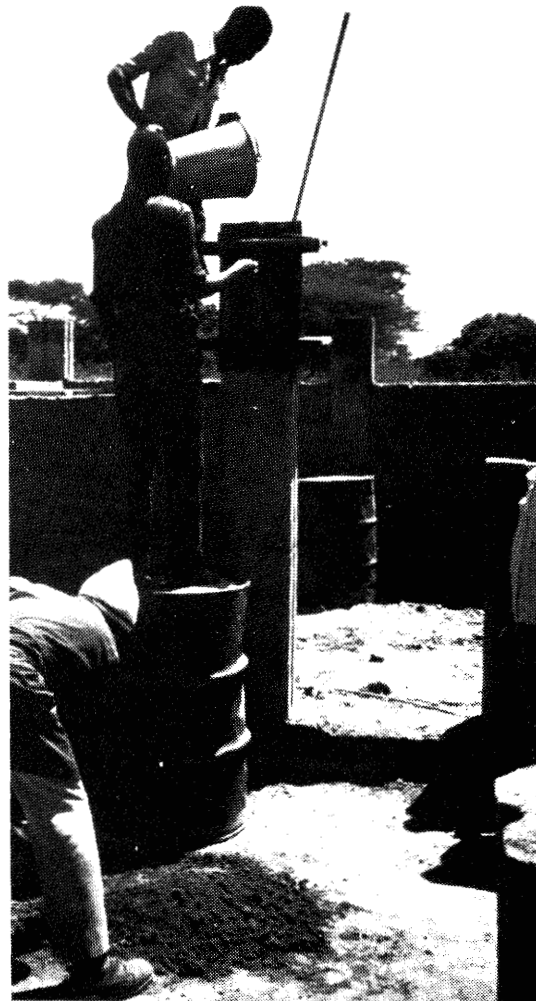
Fig. 2.6. Casting a soil-cement pillar.
