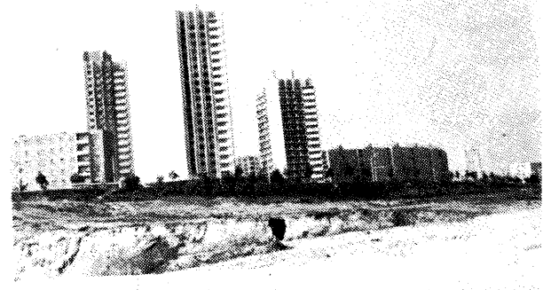
Figure VI. Minsk, Complex of 16-20-storey r.c. in-situ blocks of flats.
