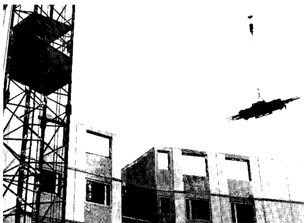
Fig. 2. Hoisting piping into the building.
