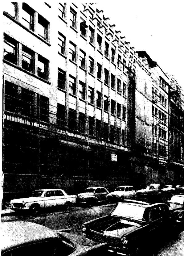
Fig. 1. EDF building, Paris. 800 window frames in stainless steel, erected in 1937, and undergoing cleaning.
