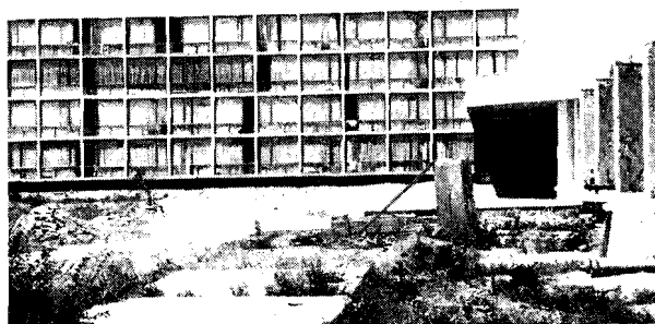
Fig. 2. Hotel built of large size panels.
