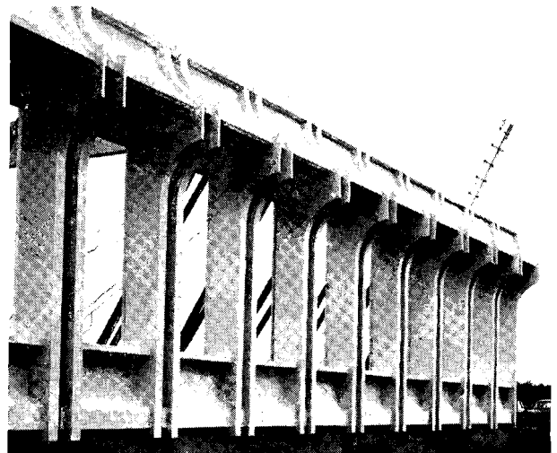
Fig. 1. Load carrying, insulated, one storey office wall panels
