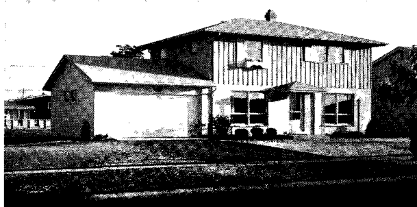
Fig. 2. Two-story UNICOM house constructed in Des Plaines, Illinois (USA).
