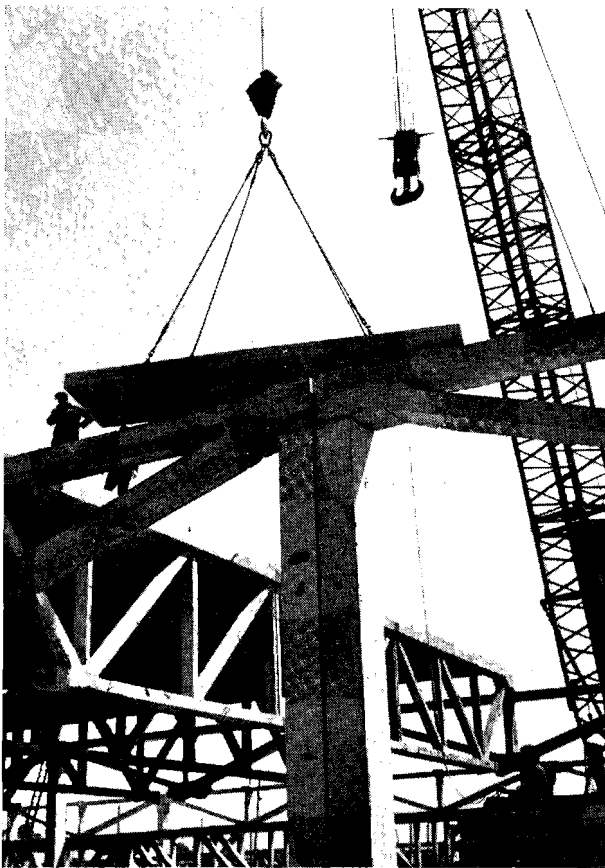
Fig. 3. Positioning a waffle-type roofing slab.
