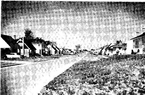
Fig. 3. Typical speculative housing development.
