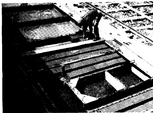
Fig. 2. COSTAMAGNA Process (France). Placing a heavy clay element in the form.
