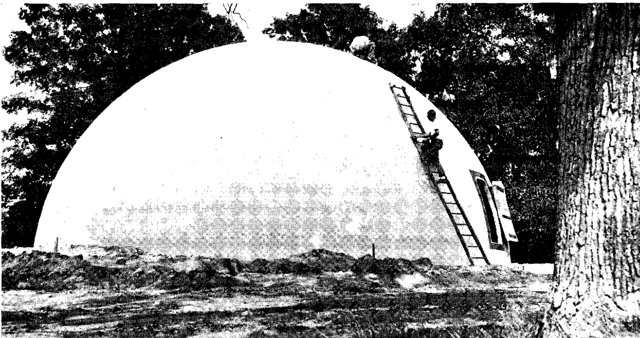
Fig. 2. Dome completed in less than 12 hours by two men and coated with latex paint and vermiculite.
