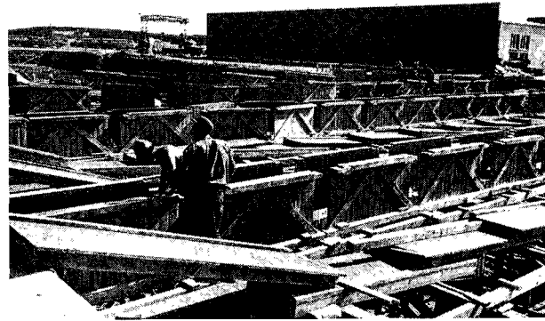
Fig. 5. Groundfloor of a large industrial hall constructed with load carrying formwork sides.
