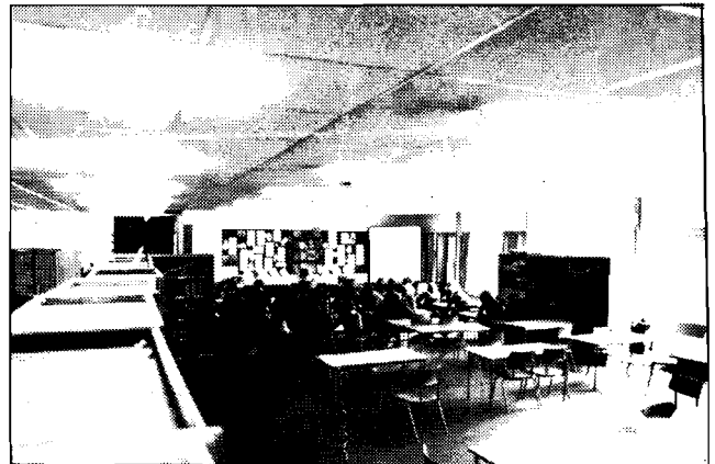
Fig 8 Photo-electrically controlled lighting installation in an open-plan school designed by the Building Research Establishment.
