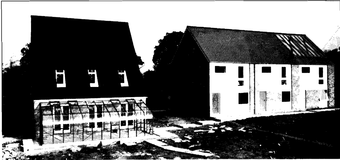
Fig 4 .View of the south face of the BRE low energy house laboratories.
