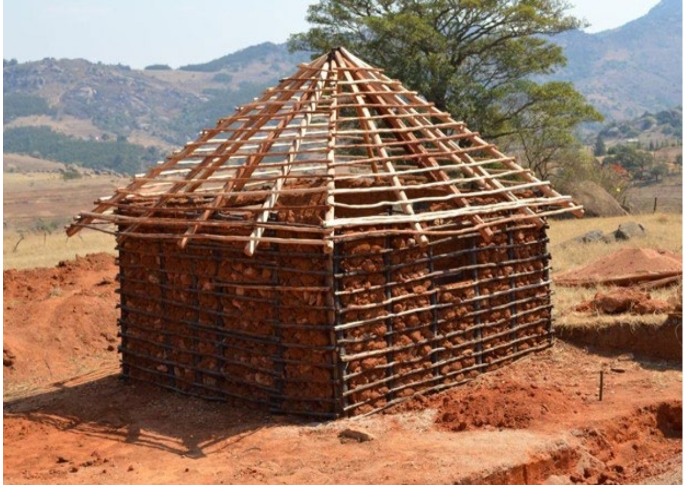
This home in Swaziland is constructed with wooden poles. The walls are filled with rocks, which will then be plastered over with mud. (Jon Sojkowski)
