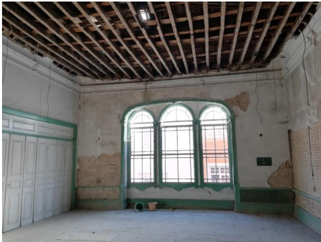
c) View of an exterior wall;
