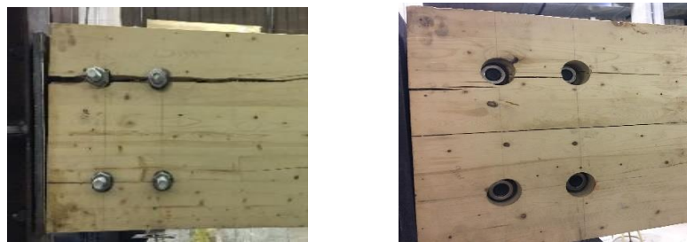
Fig. 5. Failure modes of the two beam connection configurations in ambient temperature tests; N (left) and P (right)
