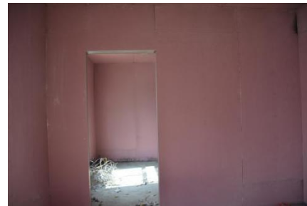
Fig. 22 Panels in fire-compartment
