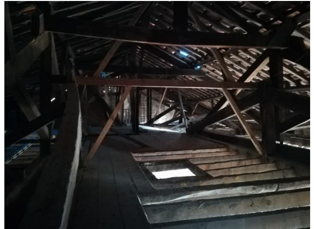
d) View of the attic timber structure
