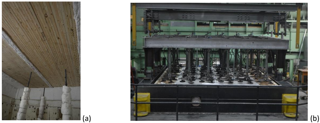
Fig. 2. Fire testing setup at the NRC: (a) view of exposed timber surface from inside furnace, and (b) distributed loading apparatus
