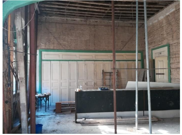
b) View of compartment walls
