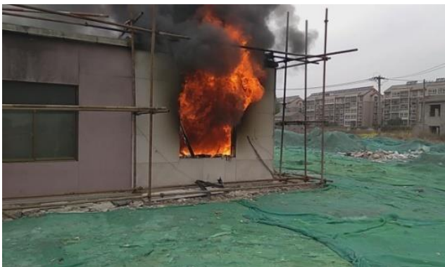
Fig. 17 Complete development of the fire
