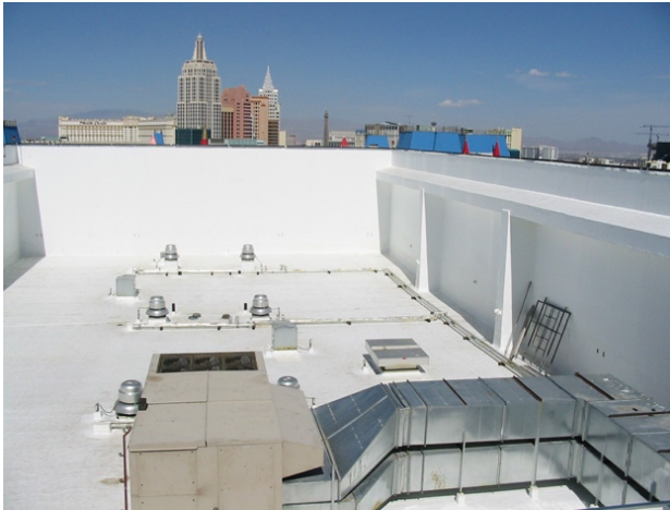
Figure 6: Reflective parapet walls
